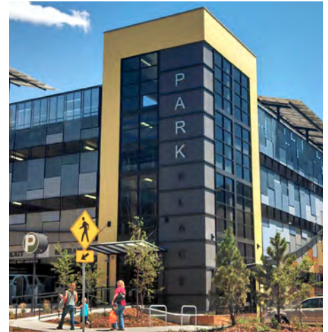
Pedestrian entries help establish a visual and physical connection between the street and an adjacent building, as shown here on a parking structure.
