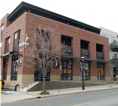
Ensure that buildings and other design features physically frame and enclose Bettie Cram and National Western Drives to enhance pedestrian comfort.
